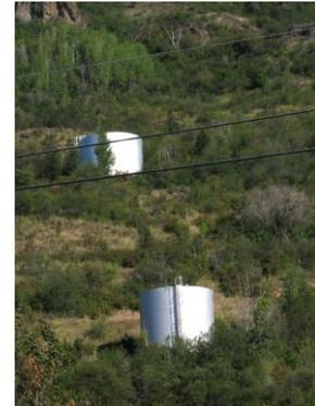
Reservoir #2 (upper) was constructed in 1979. It is also an elevated steel-finished tank consisting of one cell and has a storage capacity of 909m<sup>3</sup>. Its full water level elevation is approximately 689 metres.
