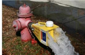
Hydrants are inspected yearly to determine the unit's ability to function properly, and to provide adequate fire protection. Village staff performs inspections such as checking the hydrant pressure, exposing any worn parts, and updating service records. In 2009, the Village began a program to include capital funding to allow for any required replacement of older fire hydrants. A total of two old hydrants were replaced and one new unit was added in 2020.
